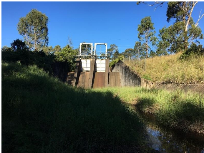
Figure 3-1 Original Grahamstown Dam spillway gates
