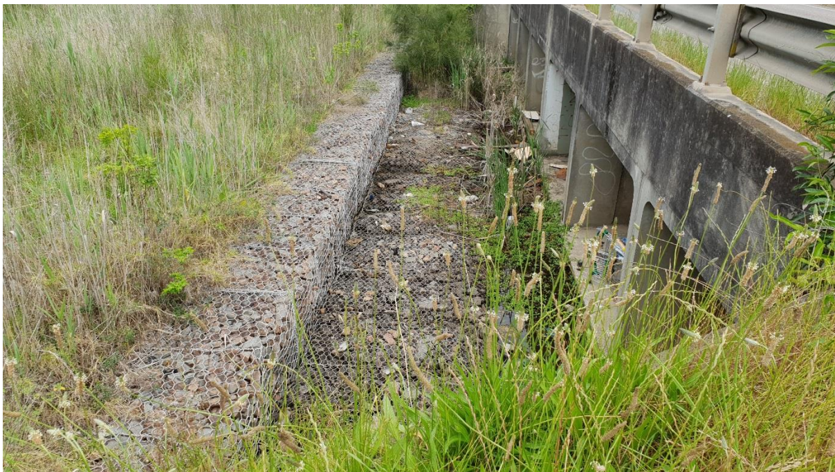
Figure 3-4 Existing gabion supported bund upstream of multi-cell box culvert
